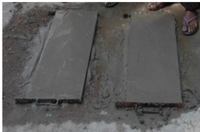
Figure 3: Casting of slab panel
