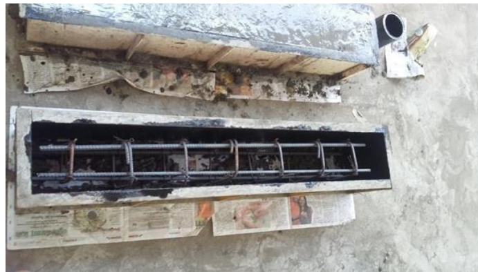
Figure 1: Casting of beam
