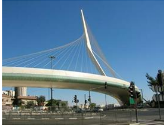
Figure 1: Side-spar cable-stayed bridge
