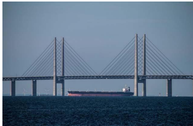
Figure 2: cable stayed cradle-system Bridge
