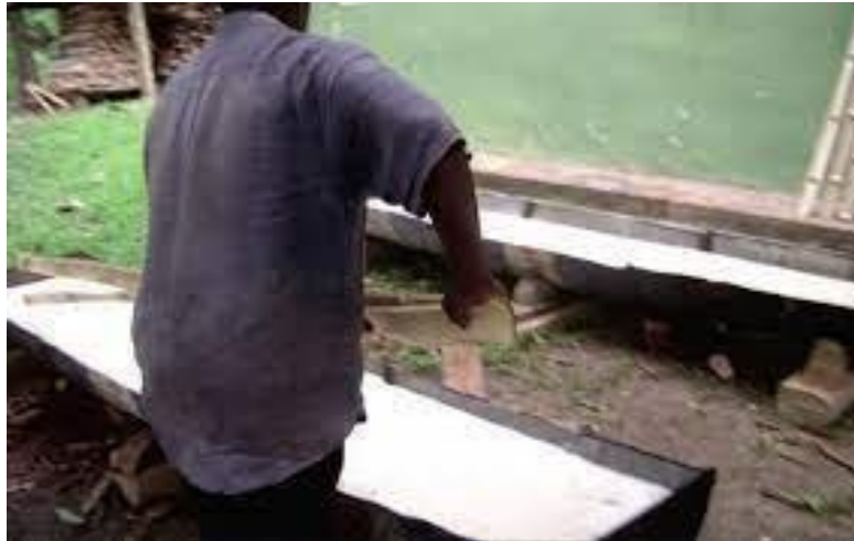
Figure 12: Bamboo treated in boric acid
